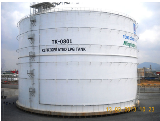
Fig. 12 Tank 2 after construction (Authors' photo)
